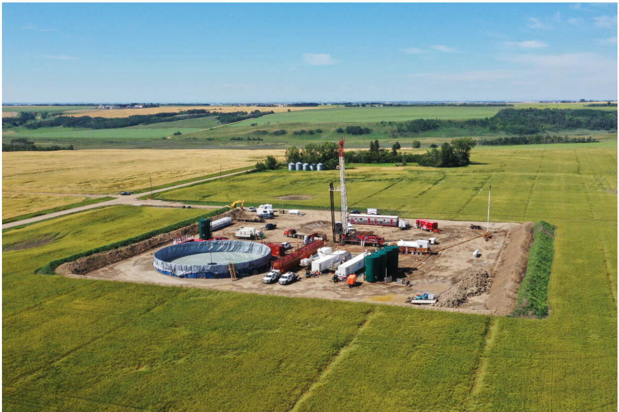
Figure 3: A conventional service rig servicing a lithium well for E3 Lithium.
